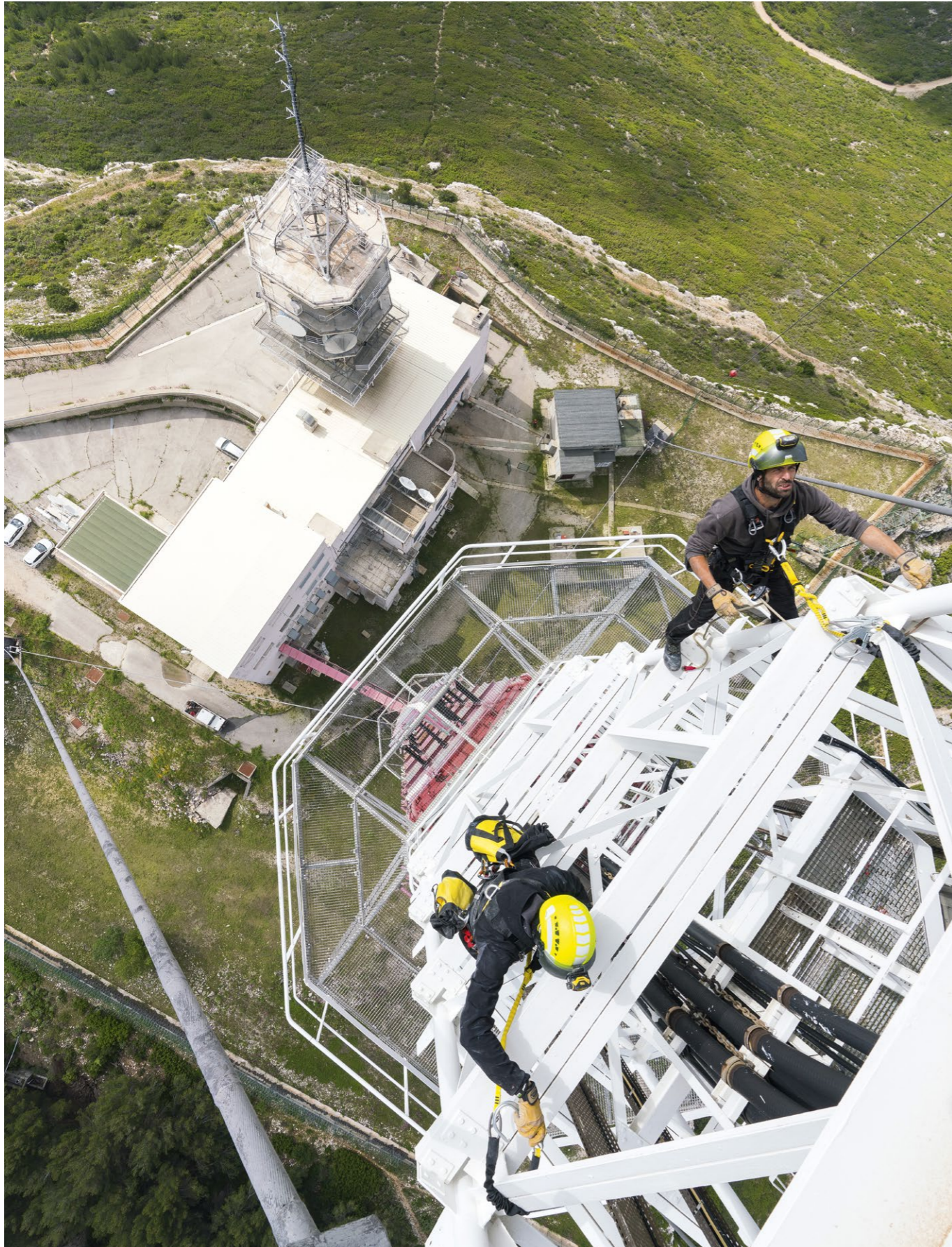
Tower inspection and maintenance, Marseille, France © 2017 Petzl Distribution - Vuedici.org - Profil - TDF
