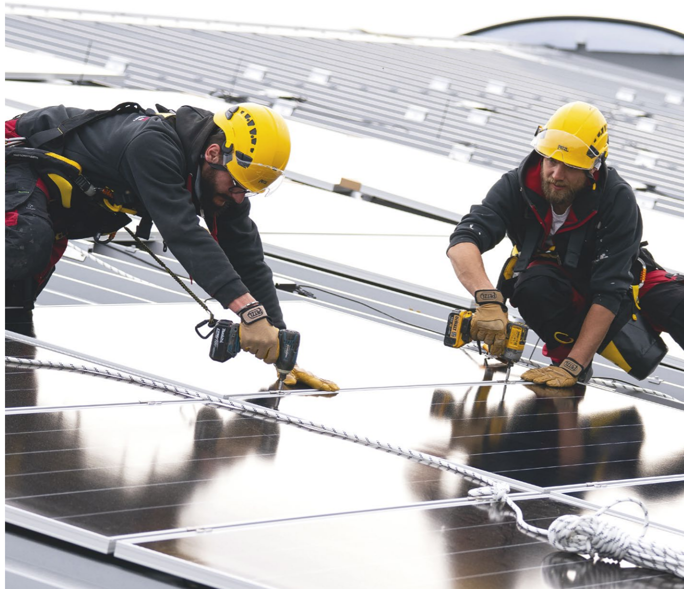
Solar panel installation, France © 2022 Petzl Distribution - Vuedici.org - Laurent Moretton
