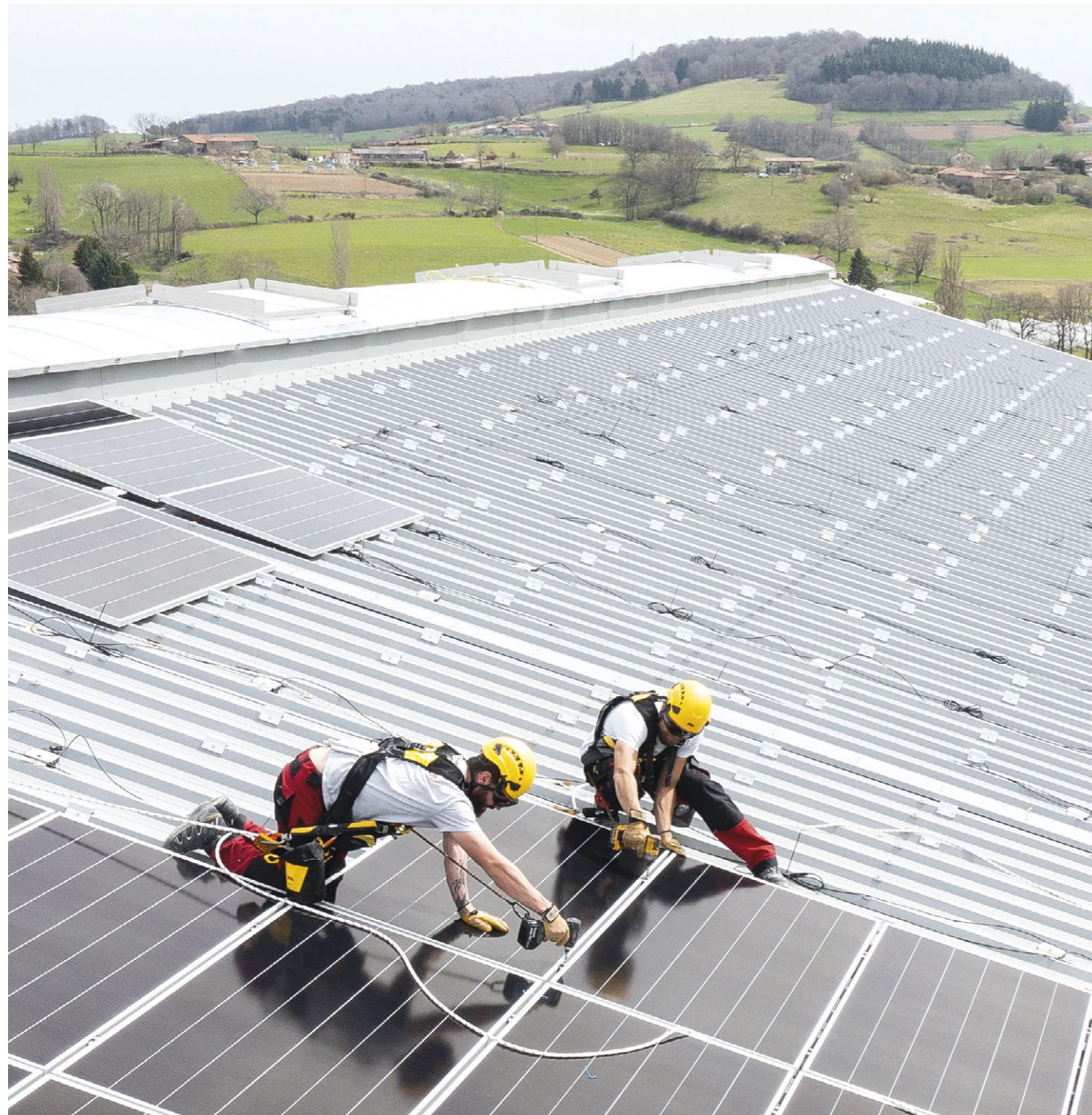
Solar panel installation, France © 2022 Petzl Distribution - Vuedici.org - Laurent Moretton
